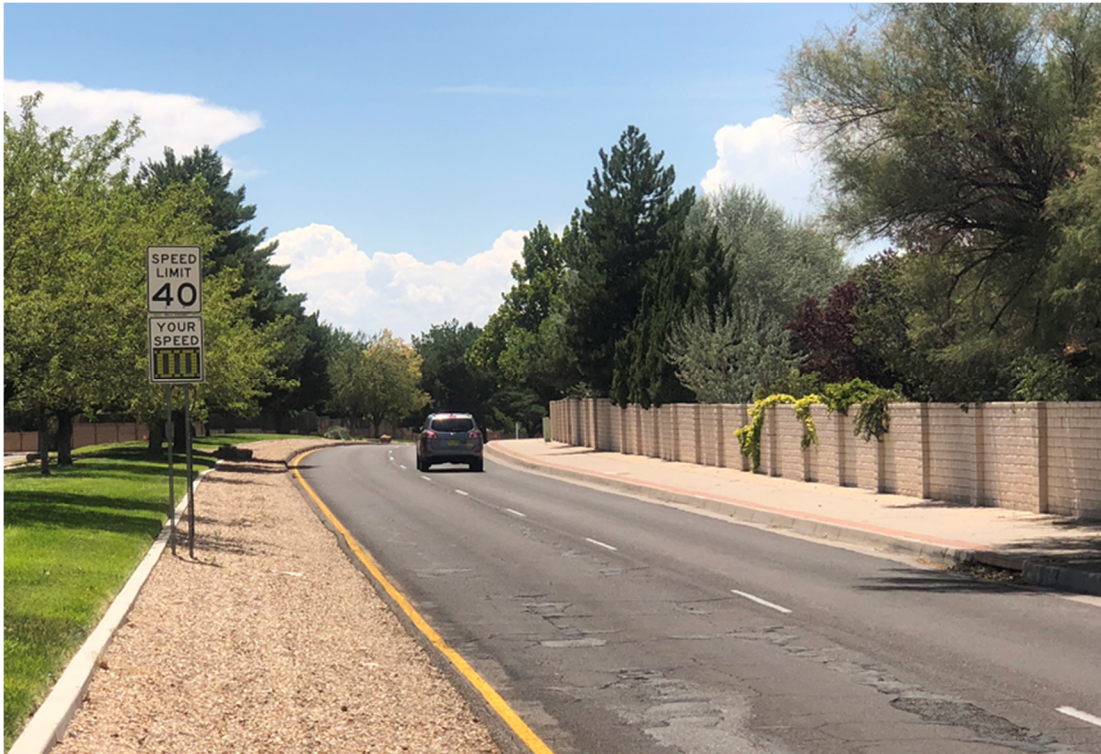
Figure 8: Academy Road Existing Speed Radar Sign
