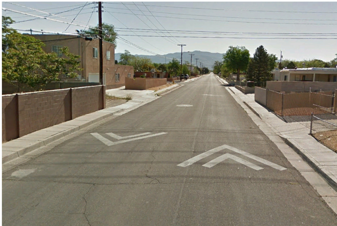
Figure 5: Claremont Avenue Existing Speed Hump
